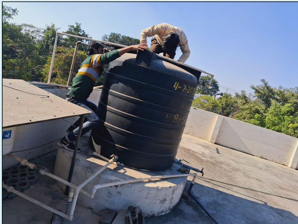
CLEANING OF TANKS
