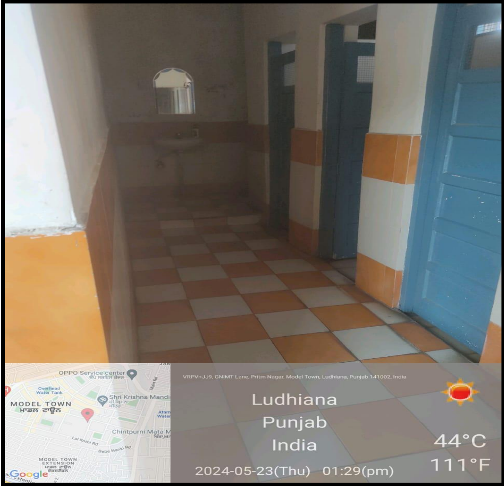
DIFFERENTLY ABLED FRIENDLY RESTROOM
